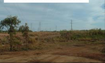
VIEW OF 66kV & 132kV TRANSMISSION LINES
