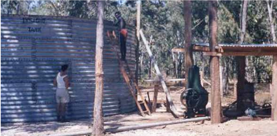
Old photo of a water tank being constructed (mission era)
