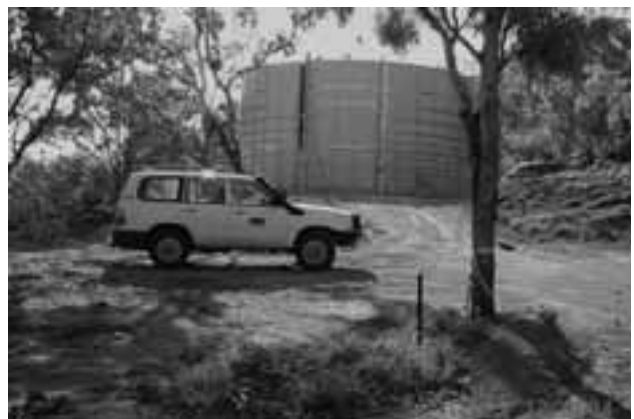
OENPELLI WATER TANK
