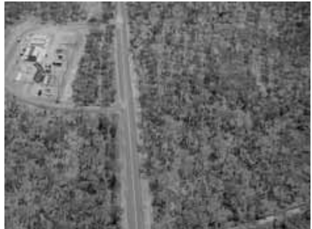
DALY RIVER POWER STATION
