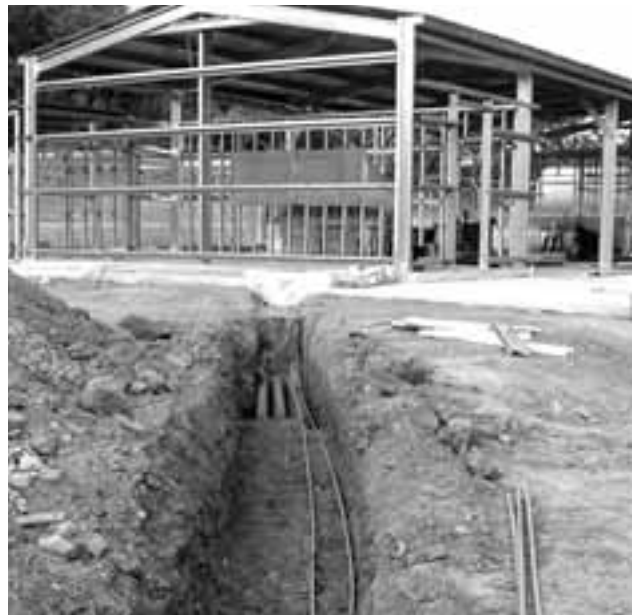
RELOCATION OF THE DALY RIVER POWER STATION
