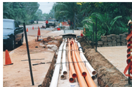
During - the trench has been dug and conduits laid.
