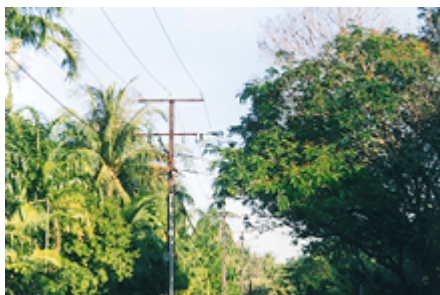
Before - a typical residential street with overhead powerlines.
