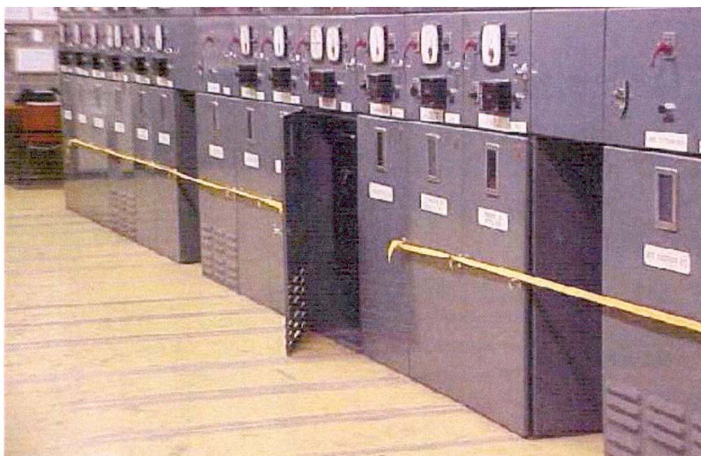
Figure 8.2.1.1 Designated high voltage access area – “Barrier out” method
