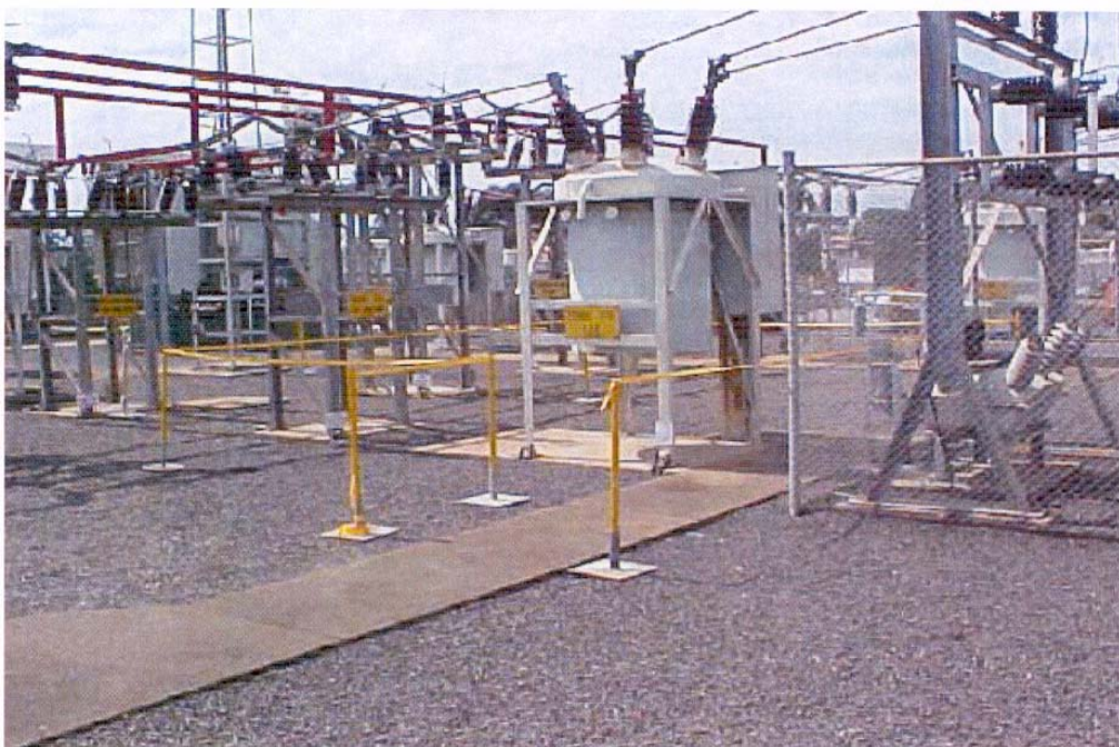
Figure 8.2.1.1 Designated high voltage access area – “Barrier out” method
